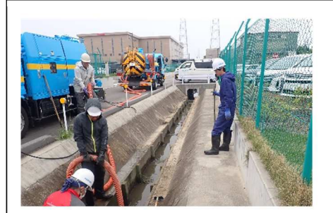
Cleaning the drainage ditch of the plant (May-2022)
